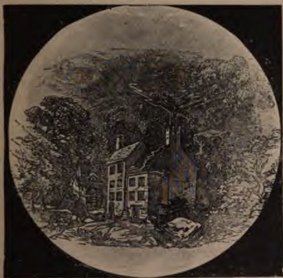
HOUSE STRUCK BY LIGHTNING, ILLUSTRATING APPARENT SIDE-FLASH FROM THE CONDUCTOR TO A RAIN WATER SPOUT.
